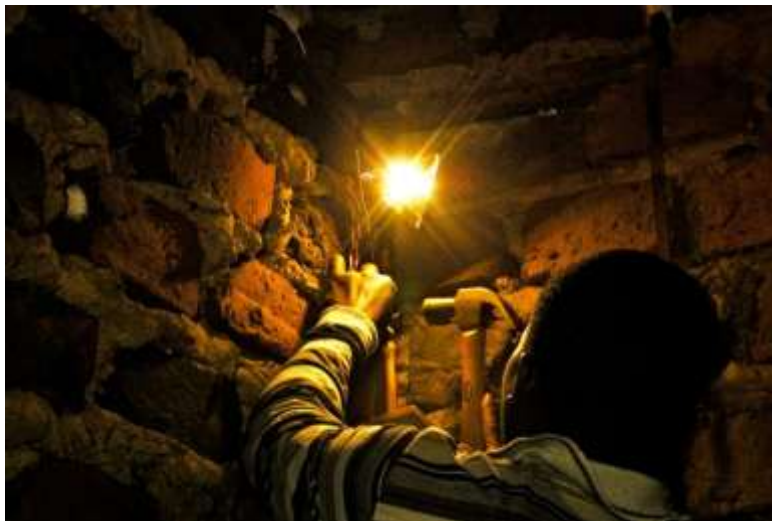
Figure 10: A solar lighting installation in progress
